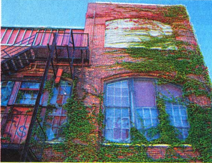
PHOTO/COURTESY DAVIS DESIGN DEVELOPMENT
